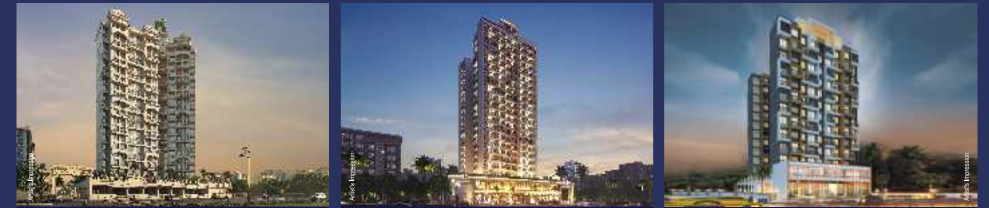
SAI SYMPHONY KHARGHAR G+27 Storeyed Tower SAI AARADHYA KHARGHAR G+22 Storeyed Tower SAI ICON KHARGHAR G+14 Storeyed Tower
